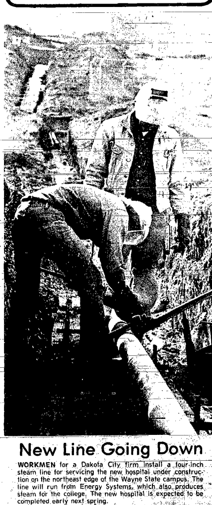
WORKMEN for a Dakota City firm install a four-inch steam line for servicing the new hospital under construction on the northeast edge of the Wayne State campus. The line will run from Energy Systems, which also produces steam for the college. The new hospital is expected to be completed early next spring.
